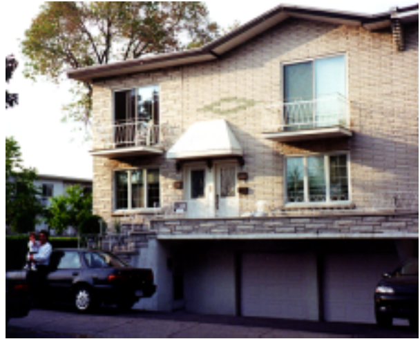
Figure 5 Case Study Building
